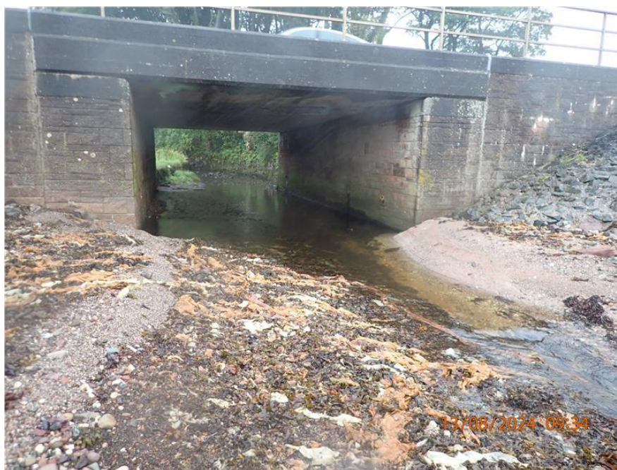
Figure 1 Site photo and condition under structure.
