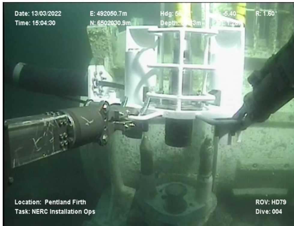
Figure 8– Wet-mate connector being positioned onto the Subsea Hub
