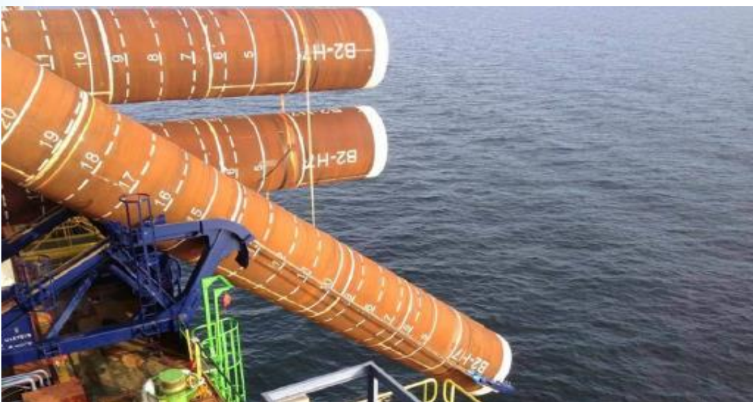
Figure 5-9: Saddle & Hook System for upending piles
