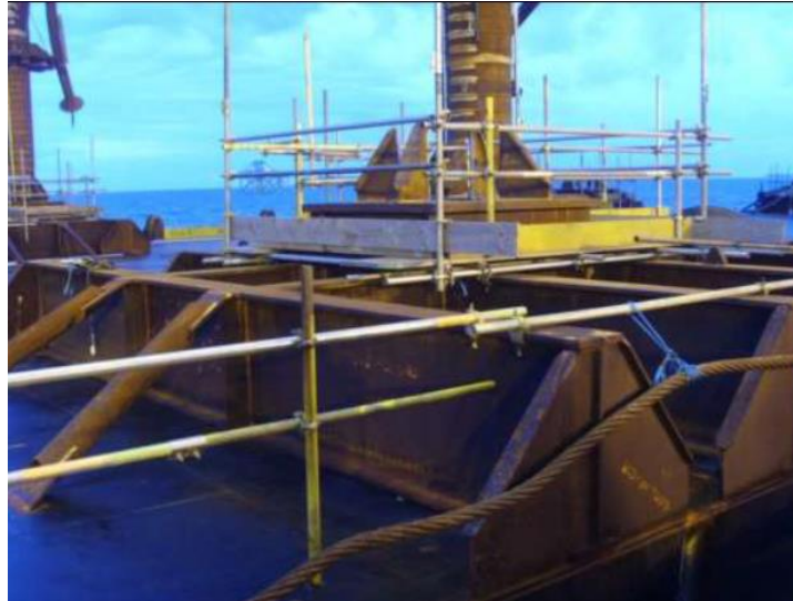
Figure 5-15: Indicative sea fastening of Jacket
