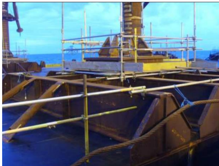
Figure 5-14: Sea fastening of Jacket
