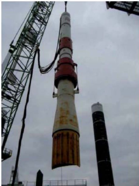
Figure 8: Typical piling hammer with follower
