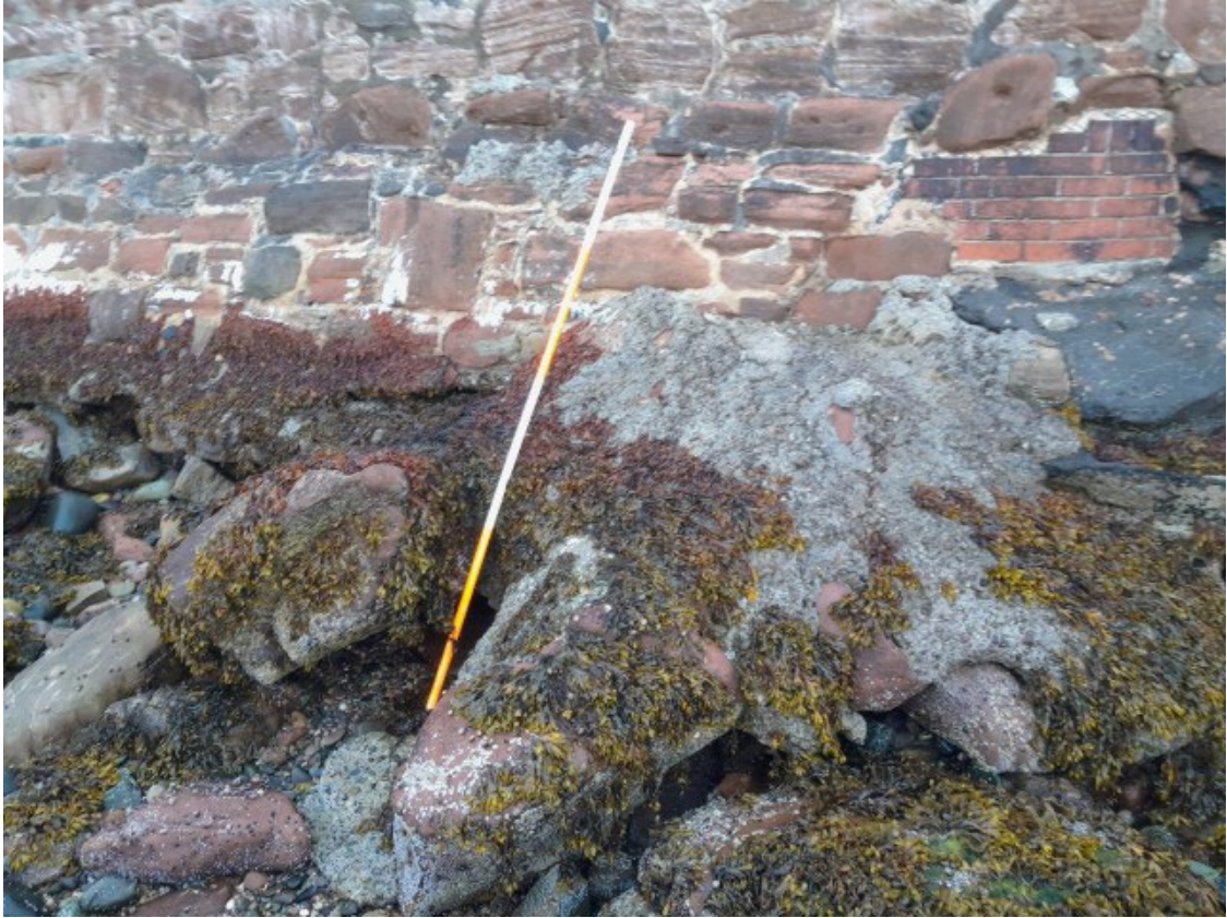
Photograph 21 - Section 3 - 9M 1411Y - mass concrete repair- 18.06.23
