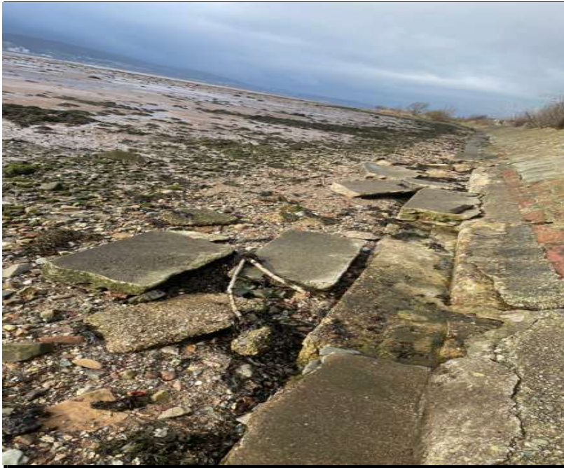
Key 1 -View along toe
