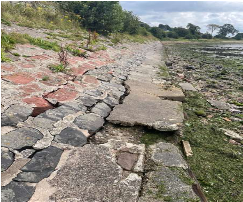
Key 2 - Section 1 - 18M 0668Y - Washout of concrete haunch along toe
