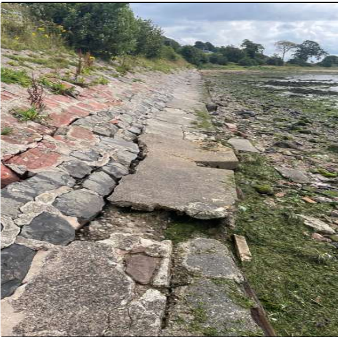
Section 1 - 18M 0668Y - Washout cracking of concrete haunch along toe
