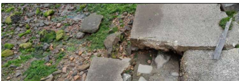
Key 2 - Section 1 - 18M 0668Y - Washout of concrete haunch along toe
