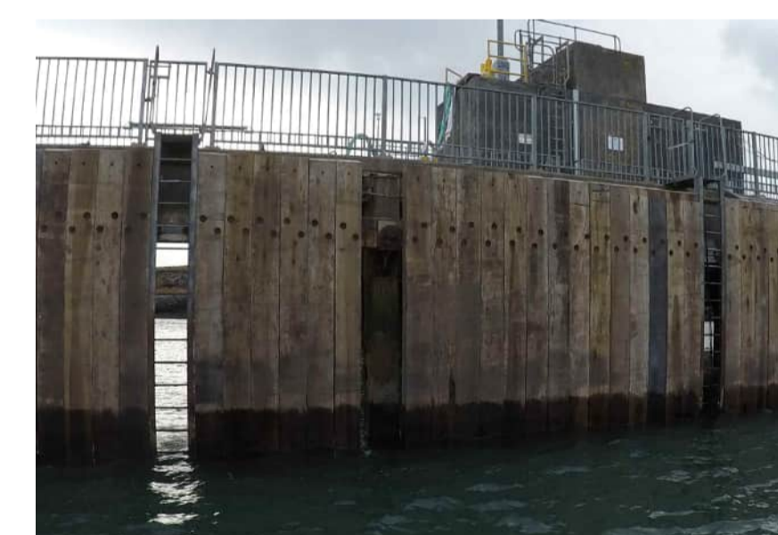
Image 7 Wave screen on Approach Pier
