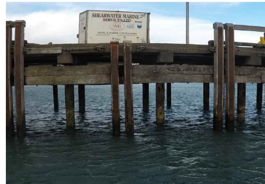
Image 3 South face of Pier
