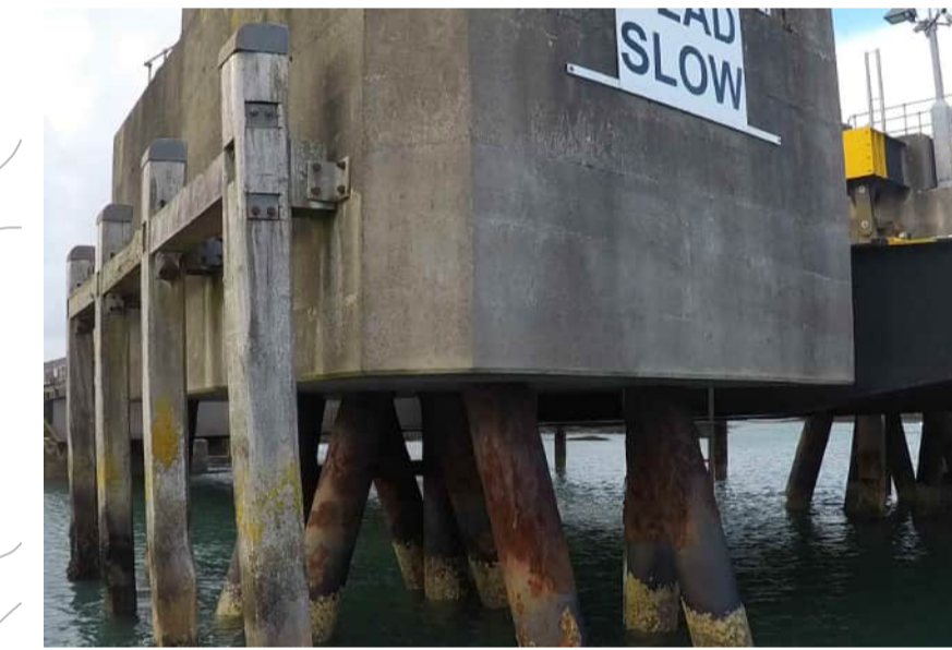
Image 6 South Lifting Dolphin
