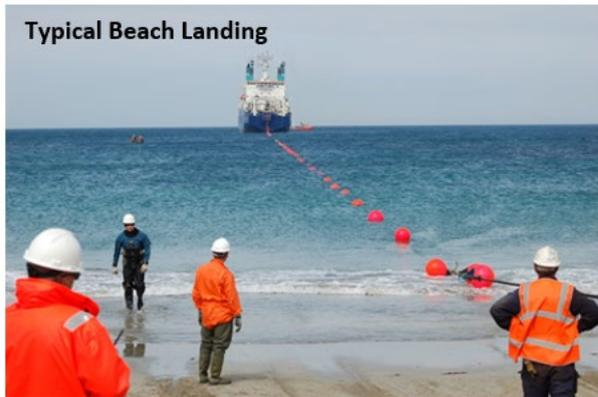
The beach manhole is typically the transition point between the marine cable and the terrestrial cable. Three existing beach manholes from Scot-NI 1 and Scot-NI 2 will be utilised, with a new beach manhole constructed at the Larne landfall.
