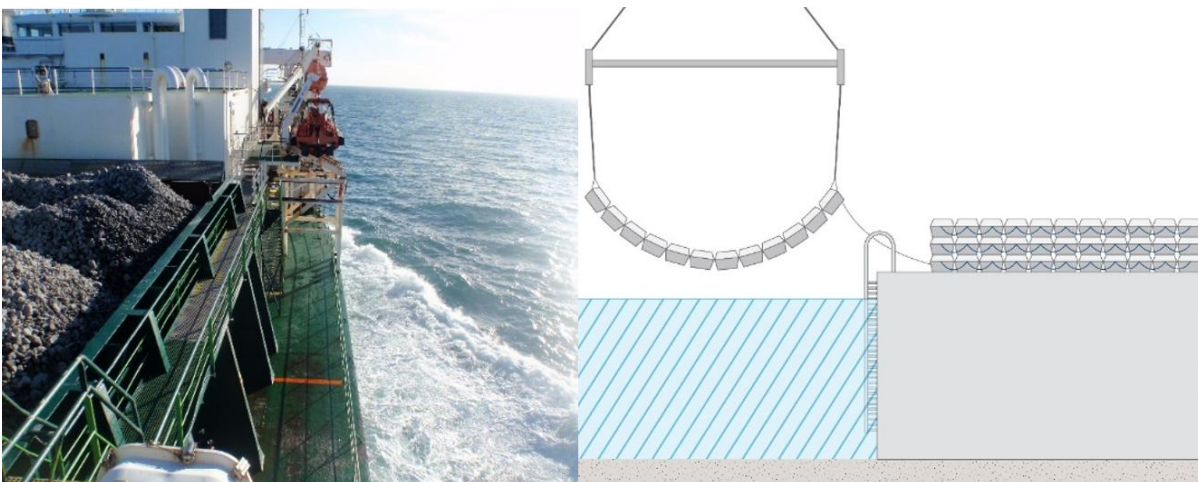
Figure 3.6: Illustrative scour protection types (Left: delivery of rock to EnBW’s Hohe See Offshore Wind Farm; Right: concrete mattresses)
