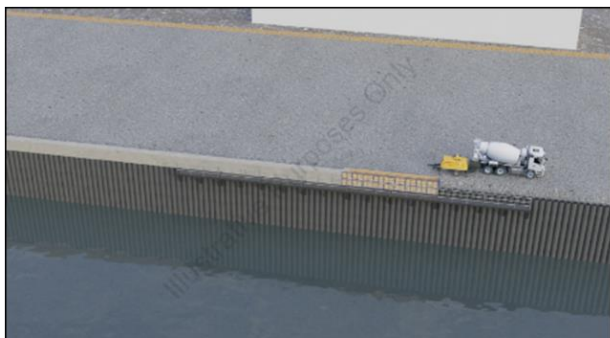
Plate 10: Coping beam installation
