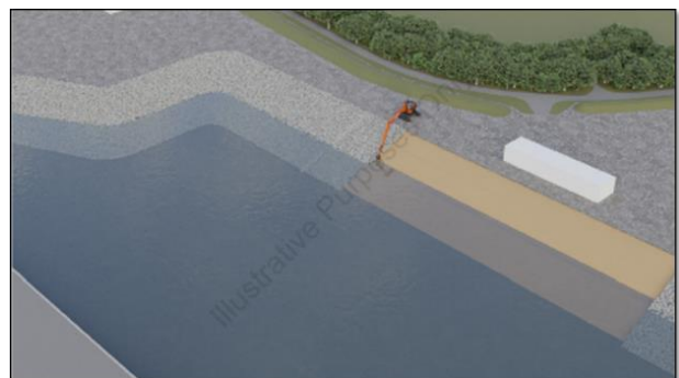
Plate 4: Rock Armour Removal
