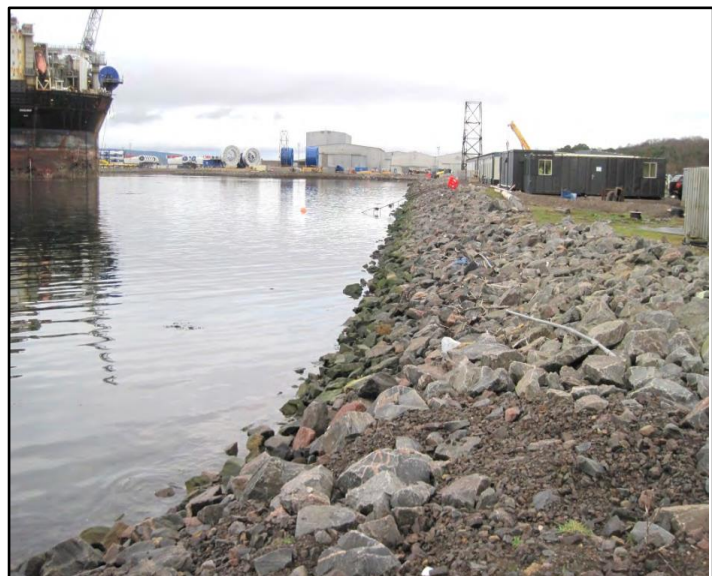
Plate 3: View north of existing Eastern Inner Dock Quay
