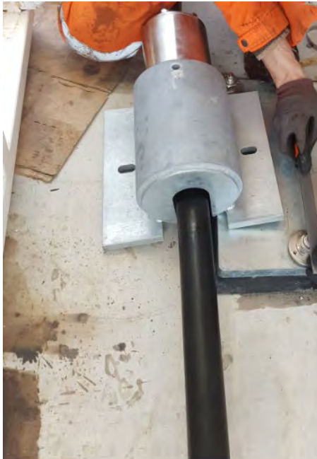
Figure 5-4 Typical subsea cable
