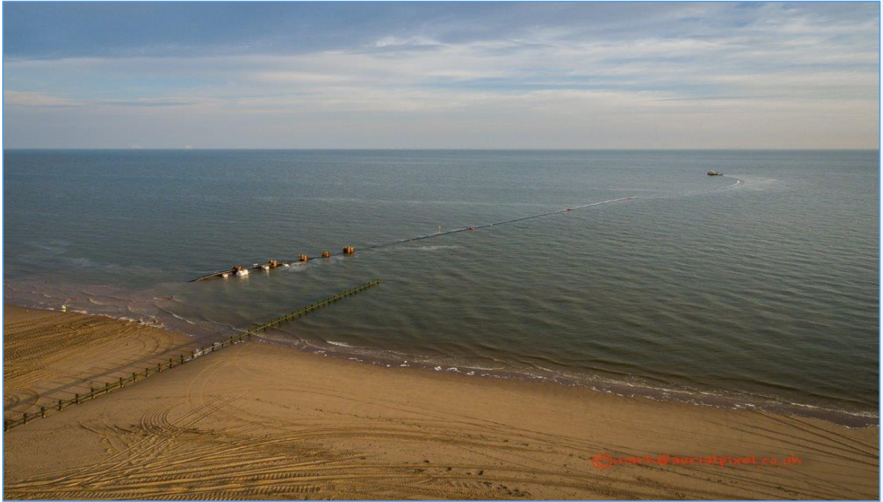
Figure 7-3: Example of HDPE duct been floated into HDD.
