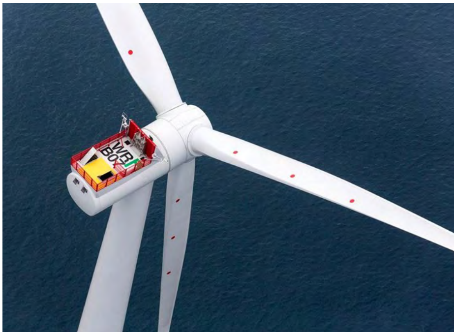
Figure 2.2 – Example of blade hover marks installed at the Westernmost Rough Offshore Wind Farm
