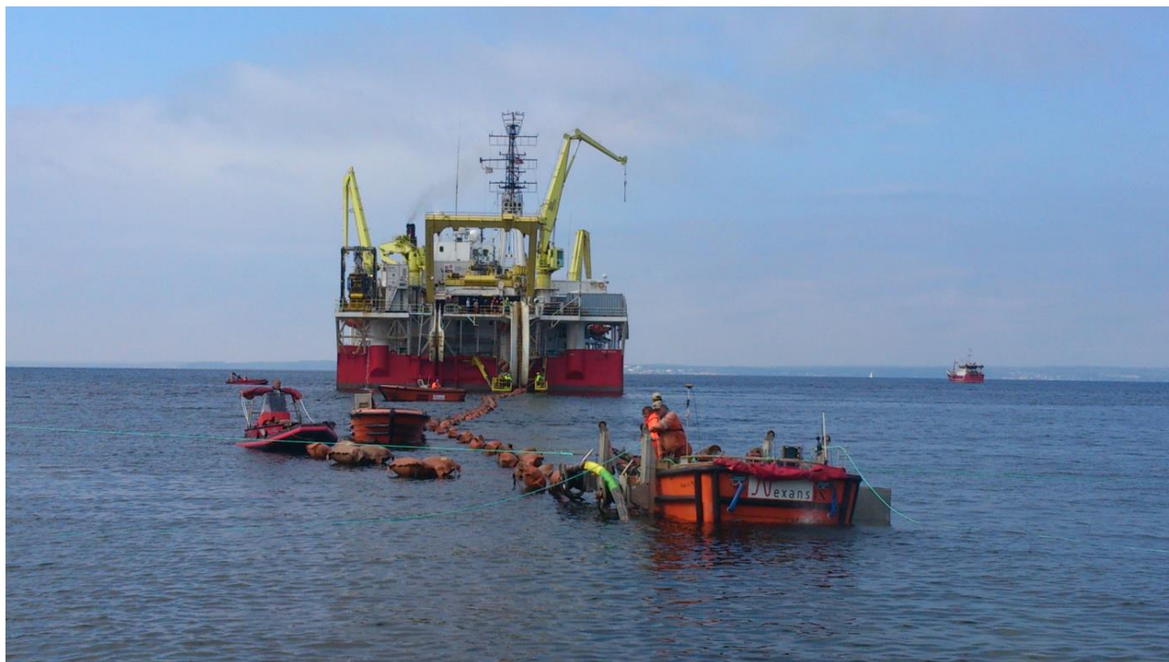
Figure 6.11: Cable floating operation (source: Nexans Consent Requirements – Construction Method Statement LF000009-NEX001-REP-K22-001-01).
