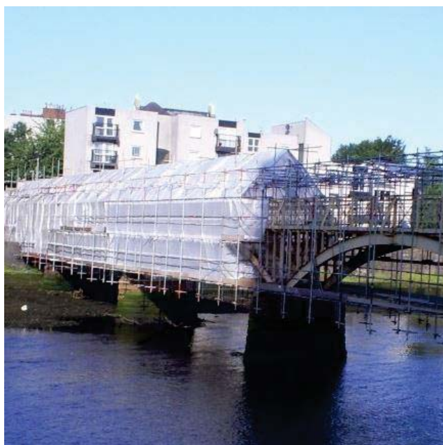
Photograph 1 – Example of encapsulation of scaffolding system set up
