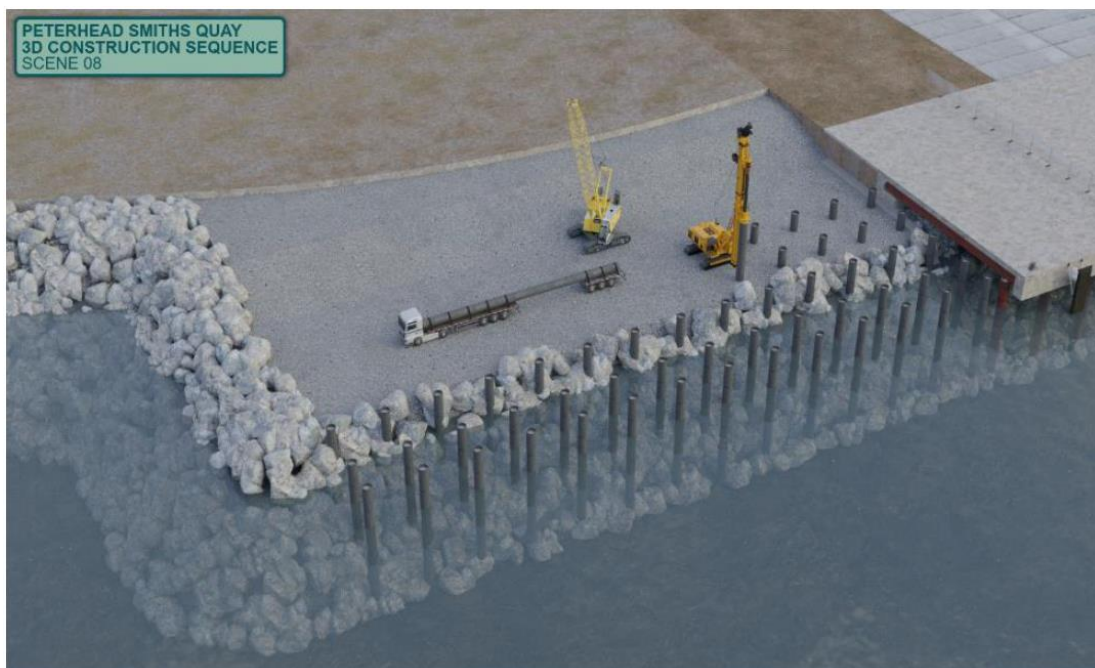
Figure 2.6 Install of pile rows A & B using land-based equipment.
