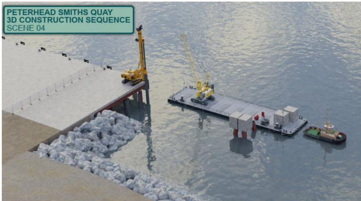
Figure 2.4 Initial pile install working from Smith Quay.
