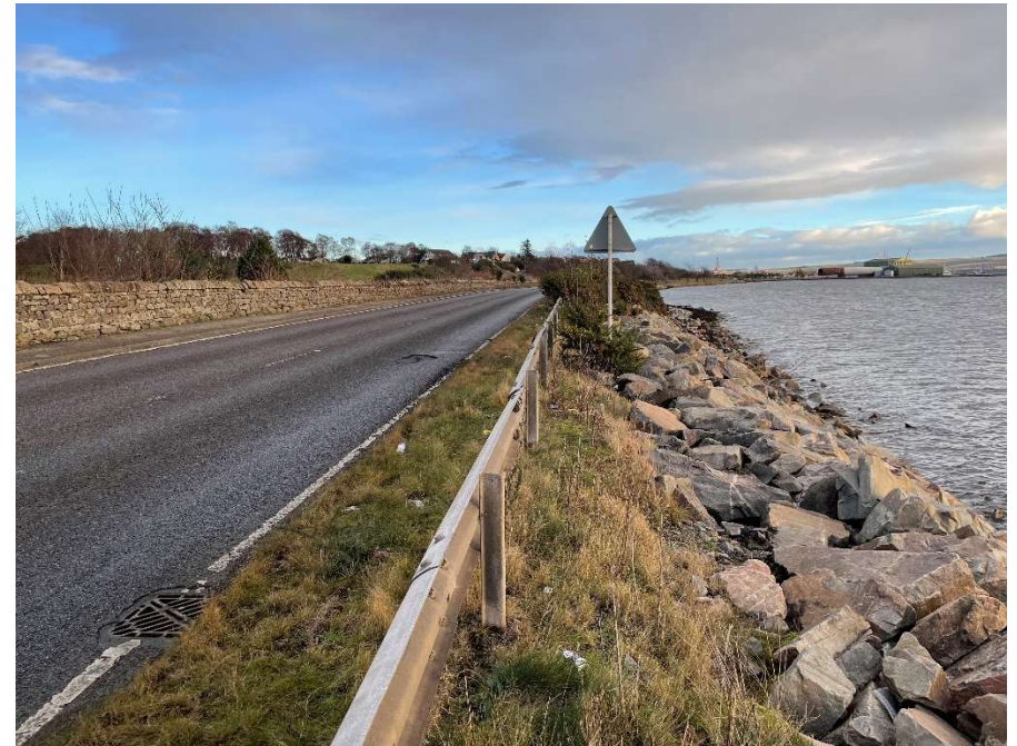
Figure 4 – Existing rock armour on right to be taken up and re-laid
