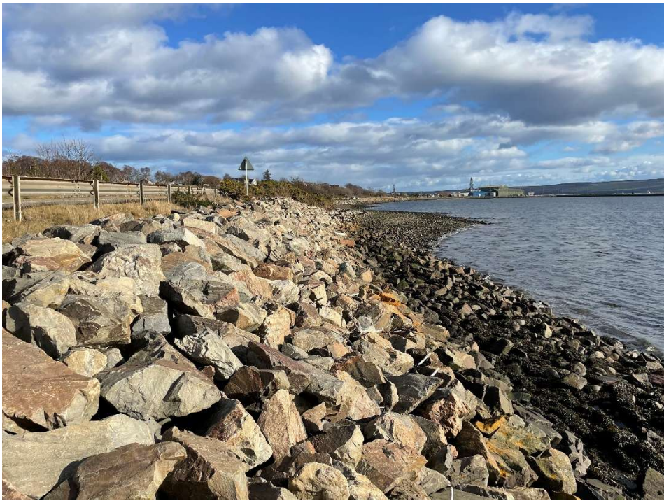
Figure 5 – Rock Armour to be taken up and re-laid
