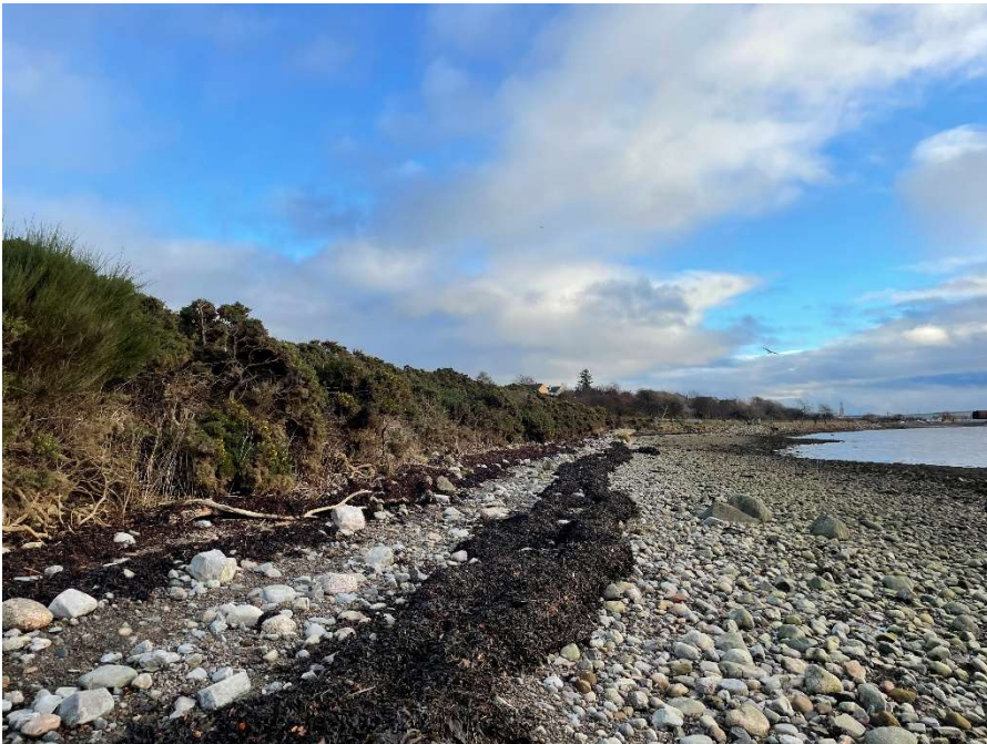
Figure 3 – Shoreline where revetment will be developed
