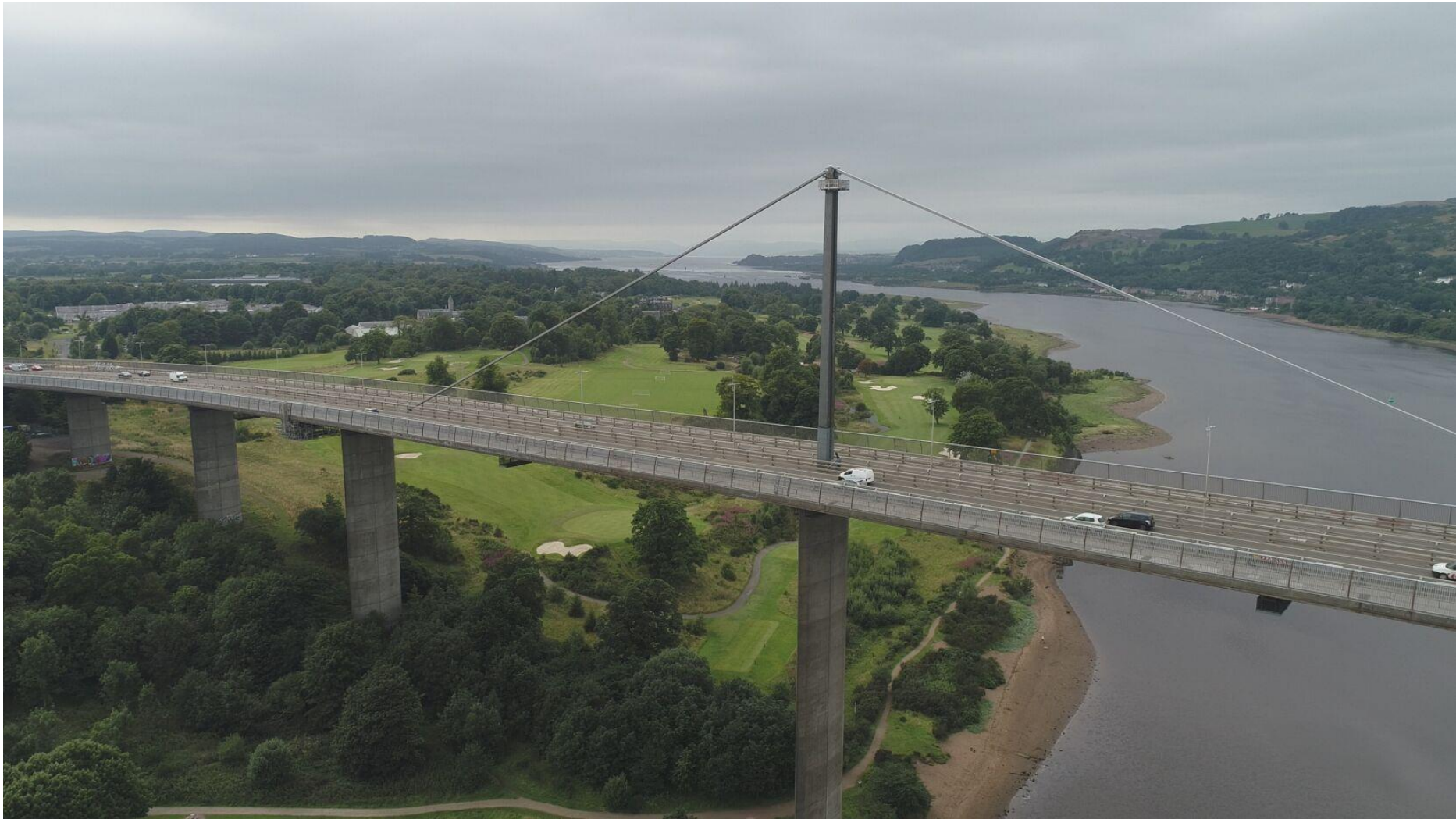
General Aerial view of Erskine Bridge (looking southwest towards Renfrewshire)
