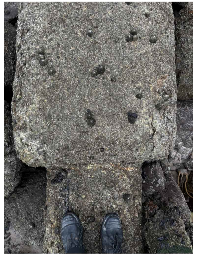
PHOTO 12 CHANGE IN CROSS SECTION OF CONCRETE ENCASURE
