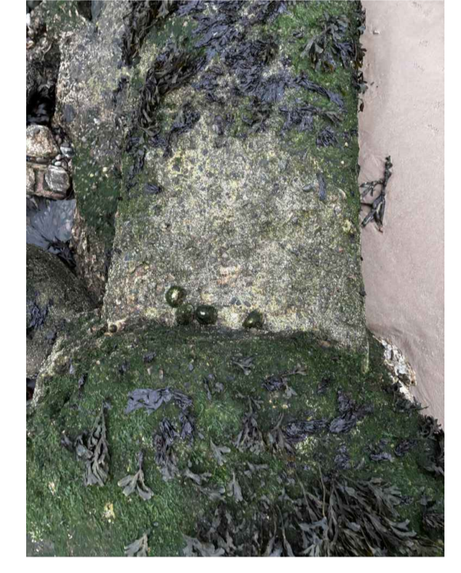
PHOTO 10 CHANGE IN CROSS SECTION OF CONCRETE ENCASURE
