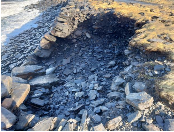
Plates 3 and 4 – damage to sea wall and wash out of made ground, 2022
