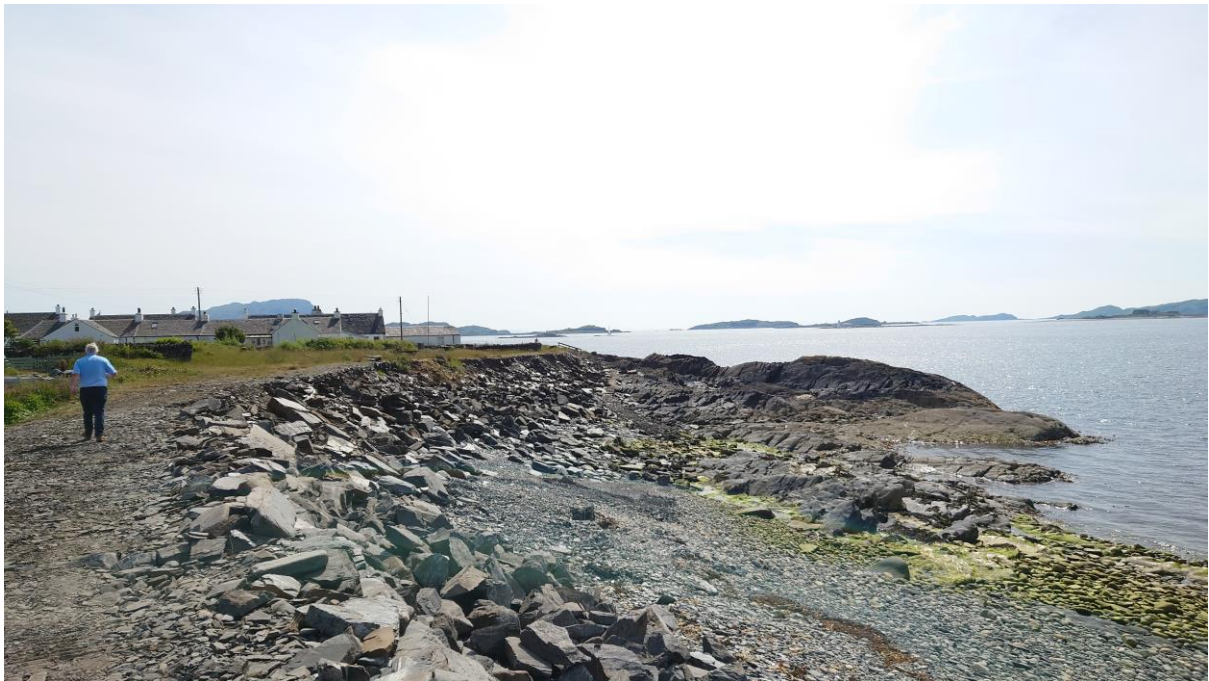
Plate 5 – sea wall with larger boulder rip rap 2023
