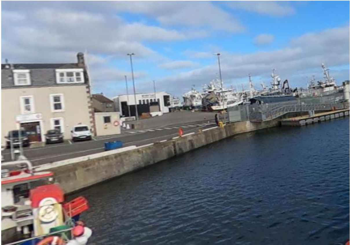
Photo 3 – General view of proposed pontoon location
