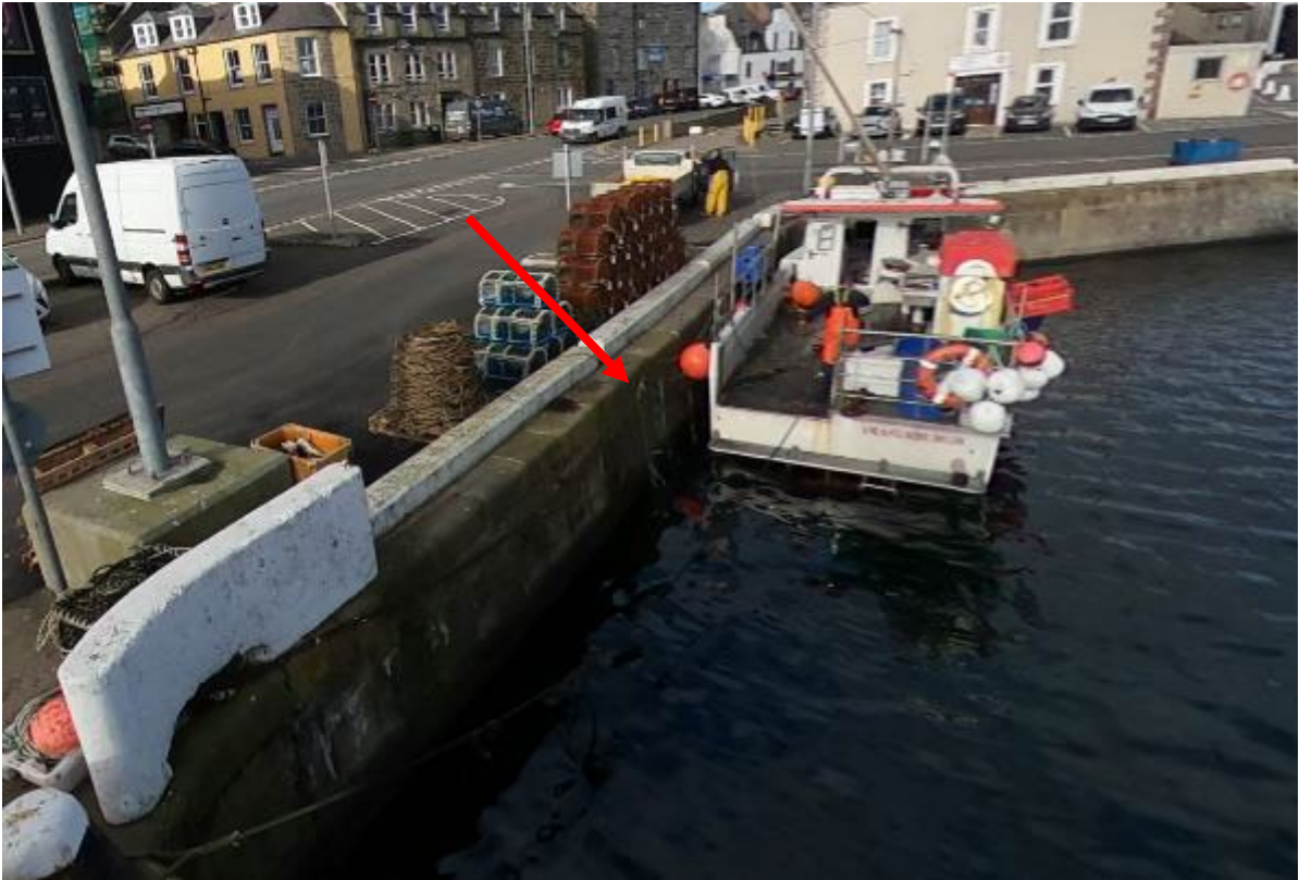
Photo 7 – Proposed location of new ladder recess and ladder
