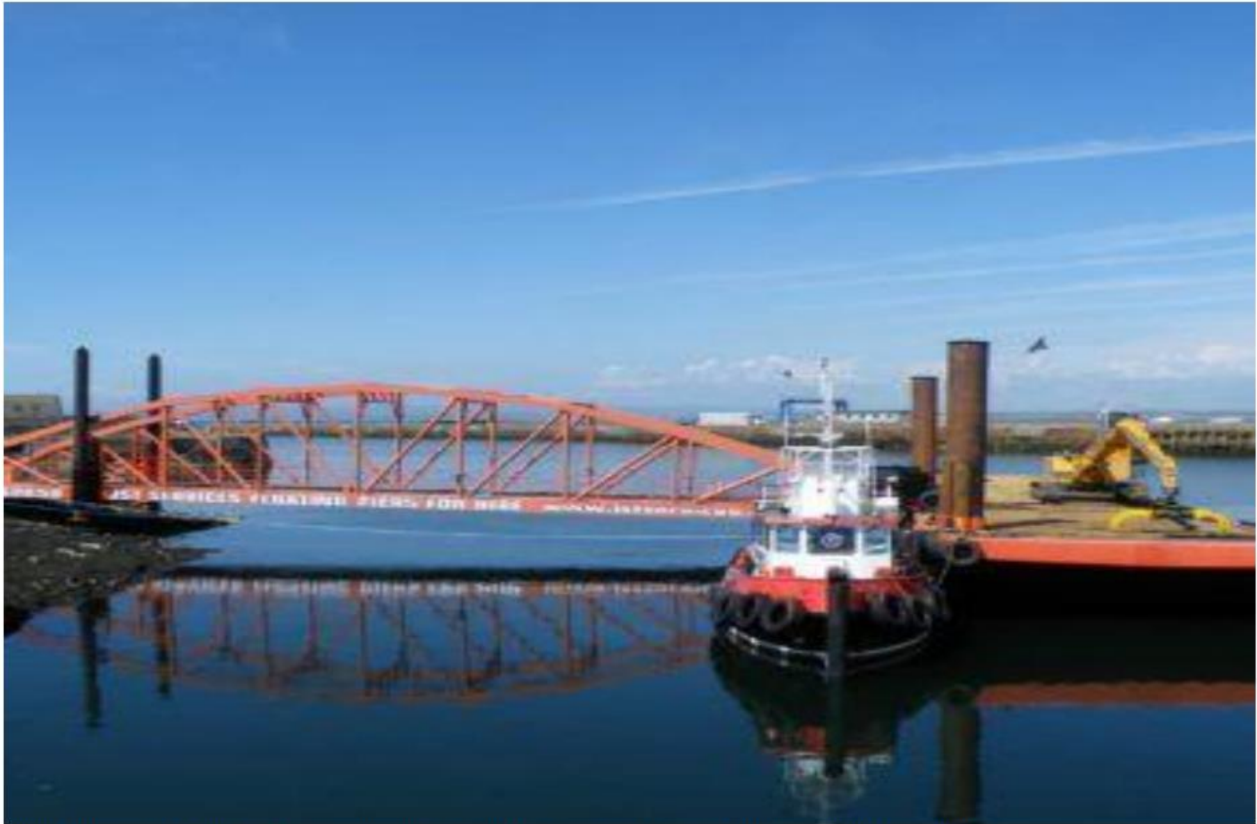
Figure 5: Image of an existing Floating Pier, before spud legs have been lowered into the seabed temporarily.
