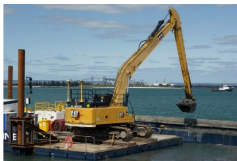
Figure 3-2 Long reach excavator on a barge
