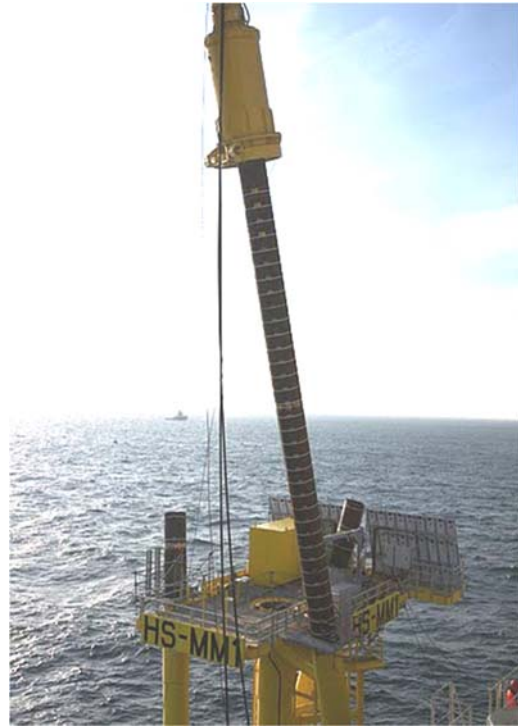
Figure 11: Photograph of post pile installation from surface
