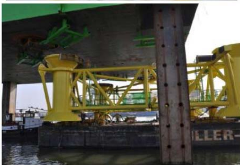
Figure 7: Transport and lowering of the PIF (from Thornton Bank II)
