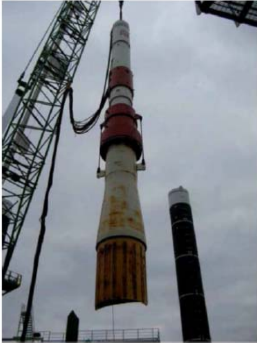
Figure 12: Typical piling hammer with follower
