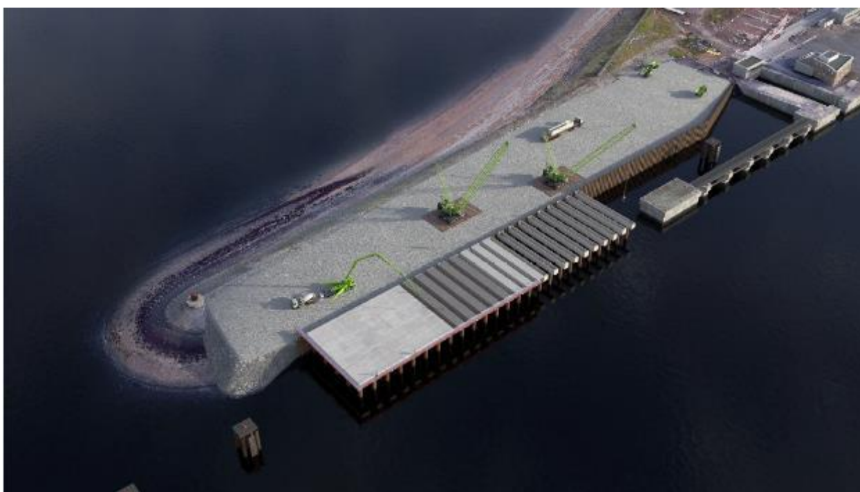
Figure 3-5 Placement of the precast beams, omni planks and pouring of the concrete deck
