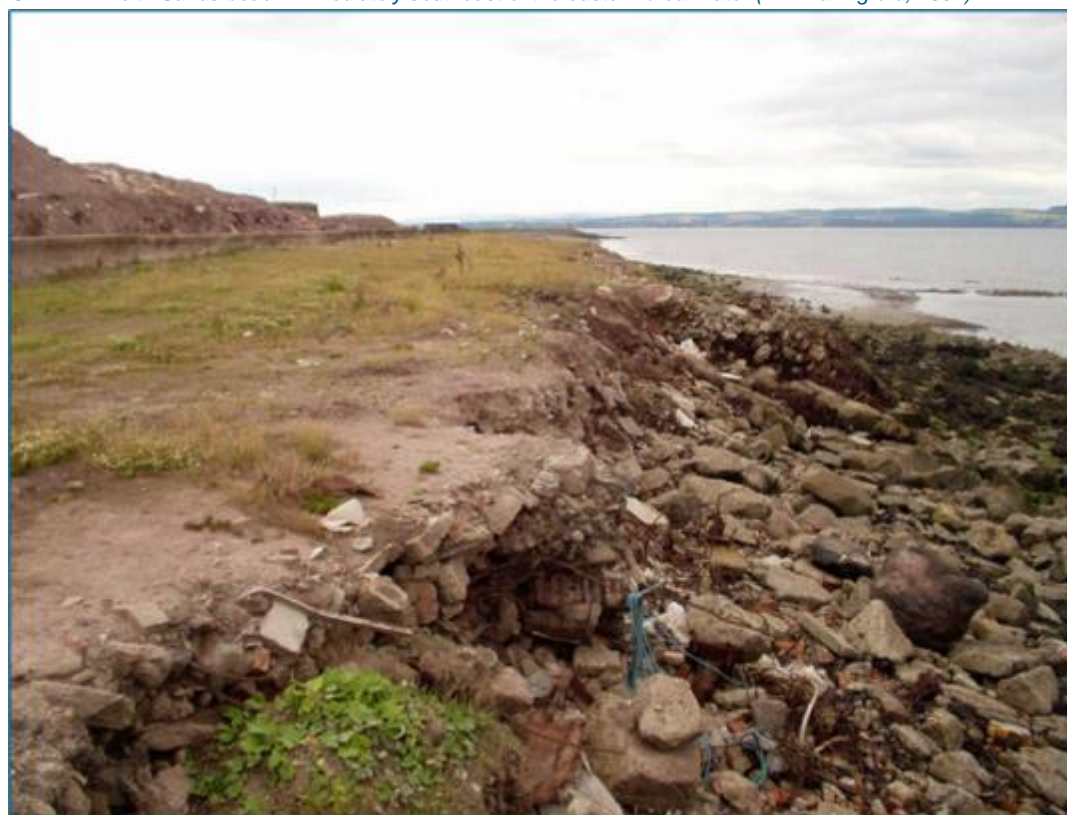
Figure 7-16 Eroding tipped building waste along Leith Sands (HR Wallingford, 2004)
