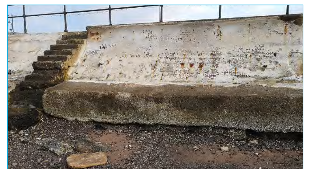
Image 6 - Wave action has exposed the toe of the seawall and caused undermining of the structure.
