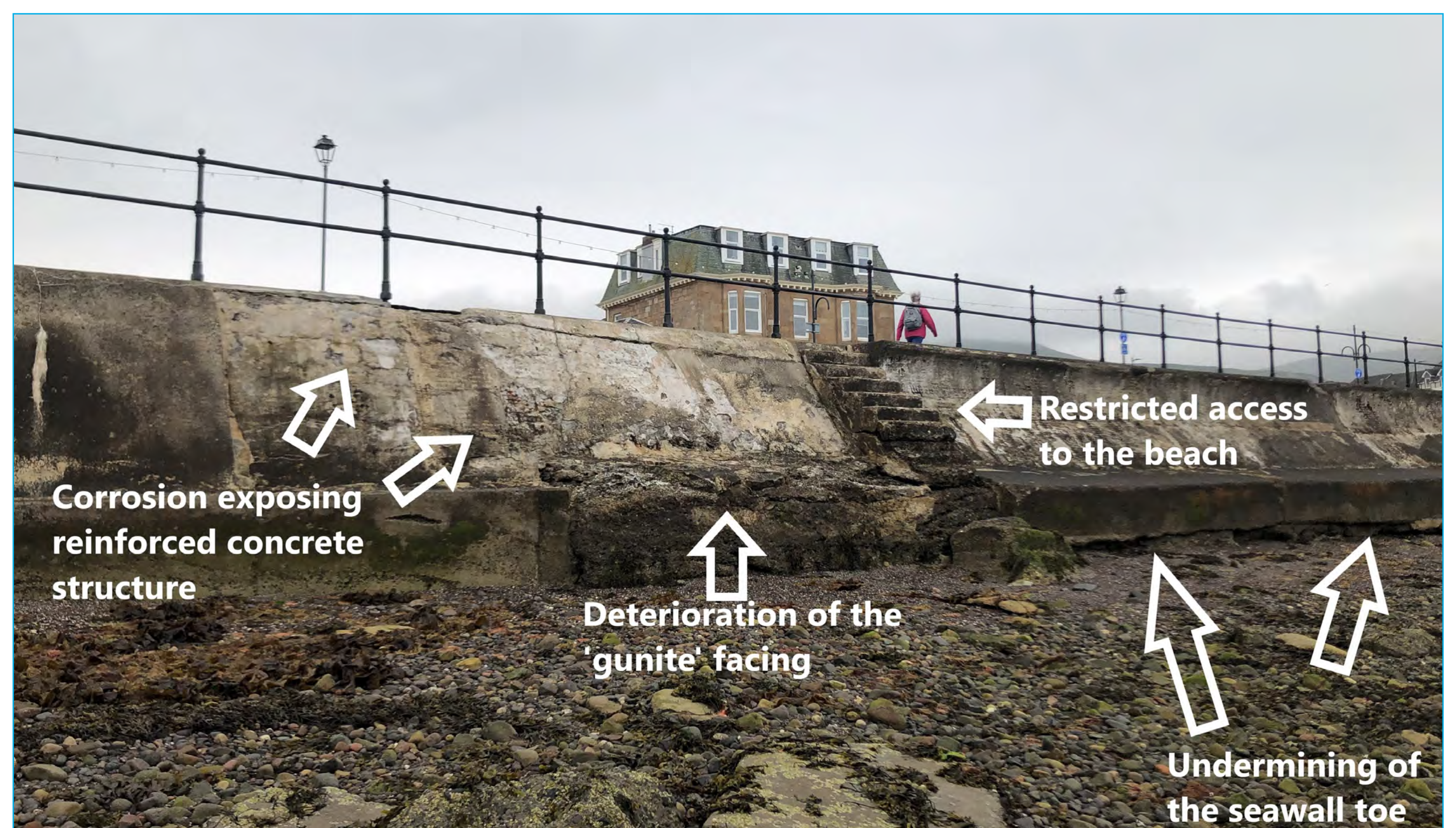
Image 7 - Deterioration of the concrete wall
