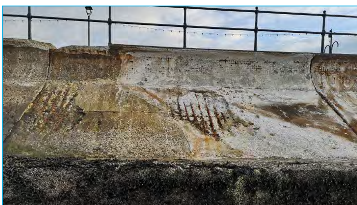
Image 3 - Deterioration of the concrete wall, exposing and corroding the internal steel reinforcement.
