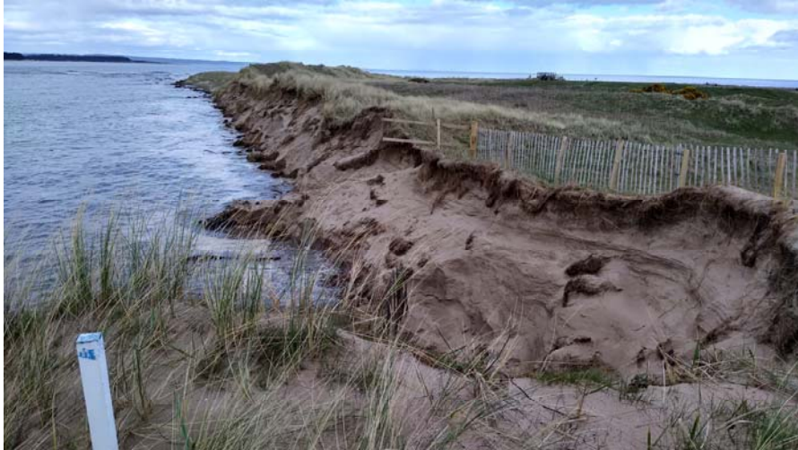
Zone of shoreline erosion, Outhead, March 2023. The area of erosion starts in the foreground in the lee of the northern end of the gabion baskets and thereafter extends northwards for ca. 120 m. Photo courtesy of Ranald Strachan.
