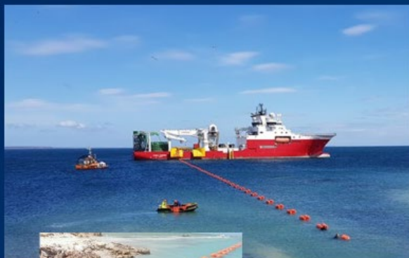
Cable Floated into beach with pillow floats
