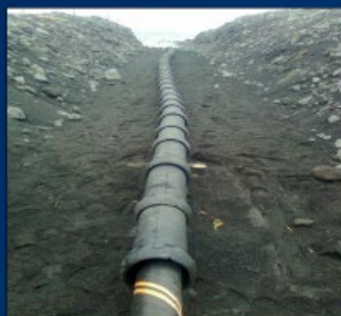
Articulated Pipe Protection at near shore and beach areas
