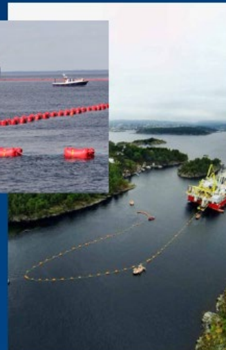
Cable Floated into beach with pillow floats
