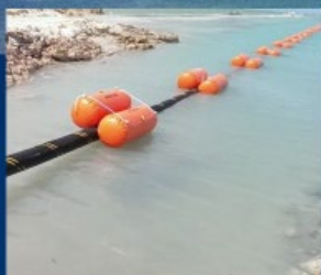
Cable Floated into beach with pillow floats
