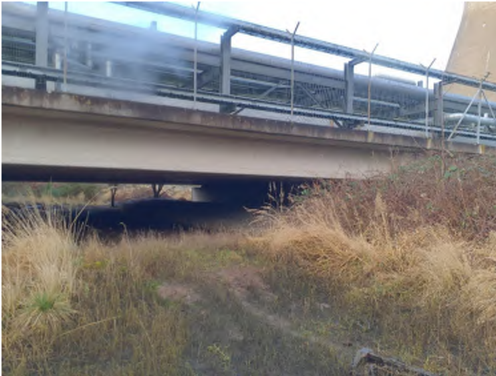
Photograph 4: View of Road 33 Bridge
