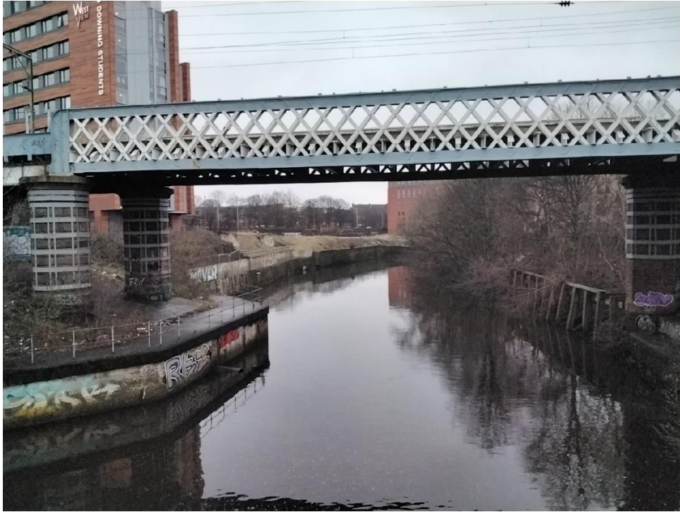
Photograph 1: Southern face of UB240/131
