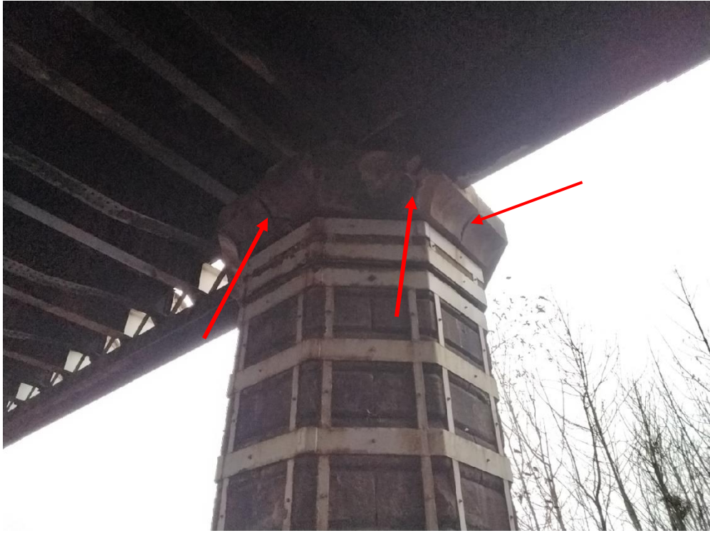
Photograph 3: Example of potential roost features on piers (red arrows)
