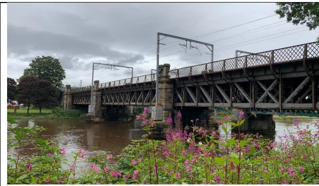
Plate 1 - Western elevation of underbridge
