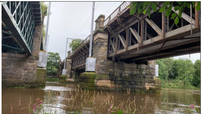
Plate 2 - Eastern elevation of underbridge
