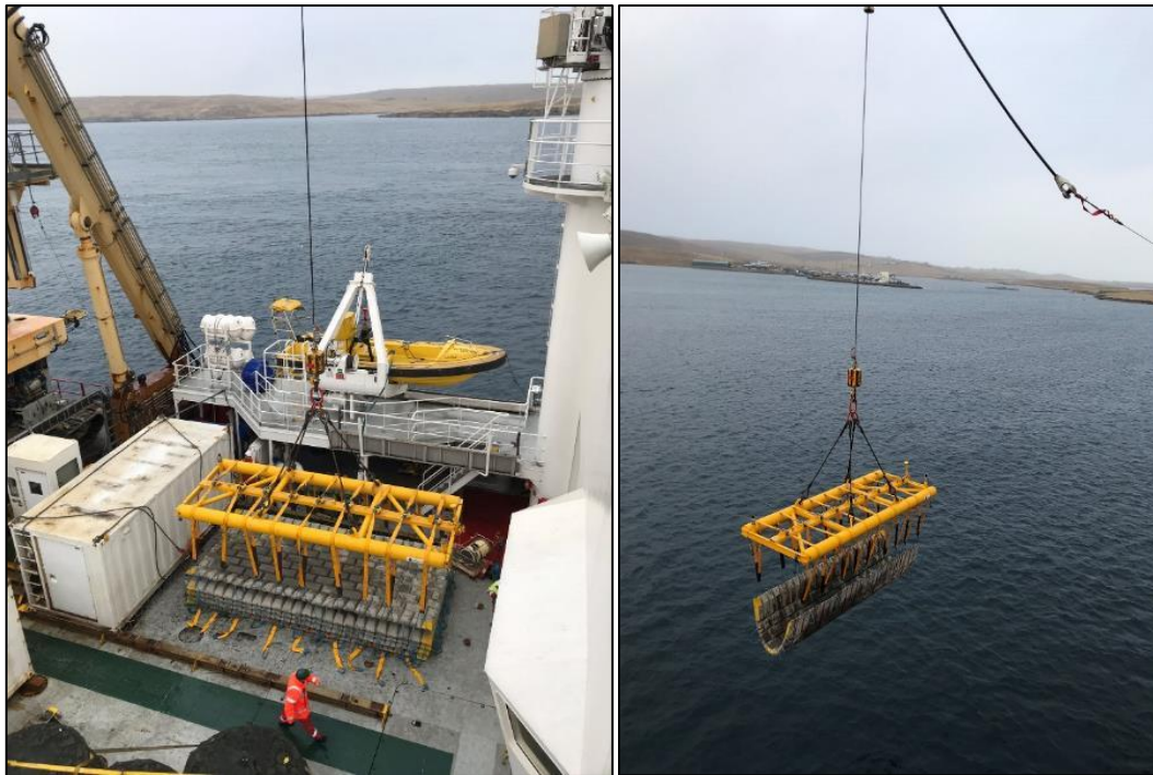
Figure 41: Concrete Mattress Deployment
