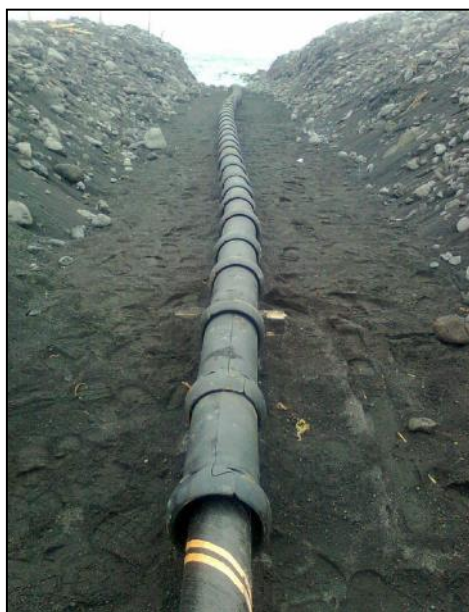
Figure 51: Example Split Pipe Installation
