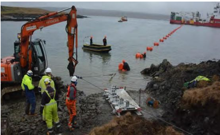
Figure 13: Example of the Beach Quadrant Layout during pull-in
