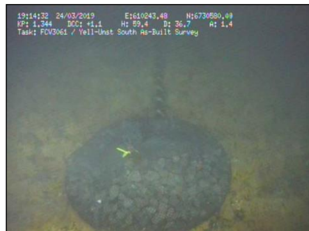
Figure 47: Rock Bag in Position Subsea
