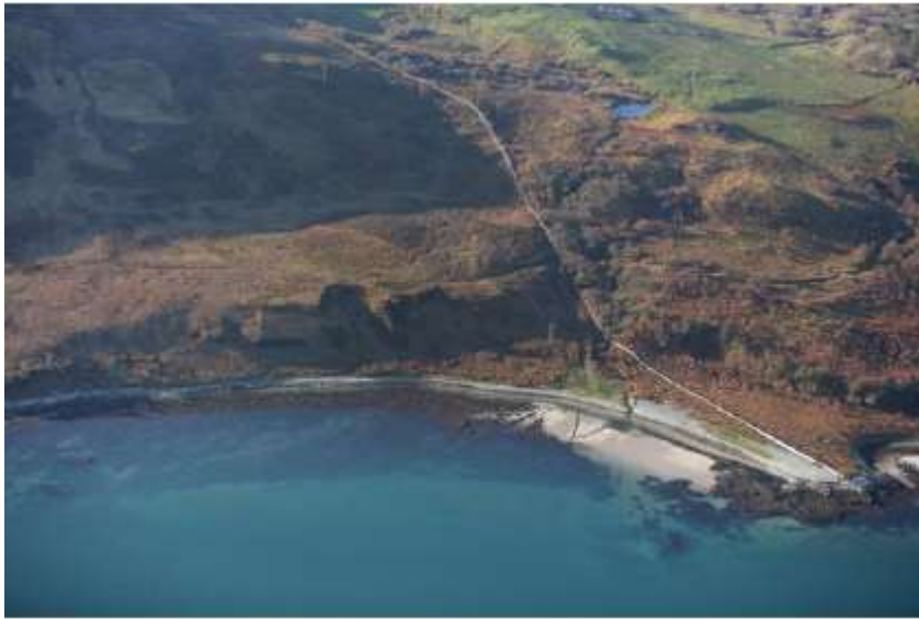
Figure 5-10 Islay landfall site
