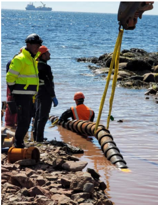
Figure 5-21 Example Cast Iron Shell Installation
