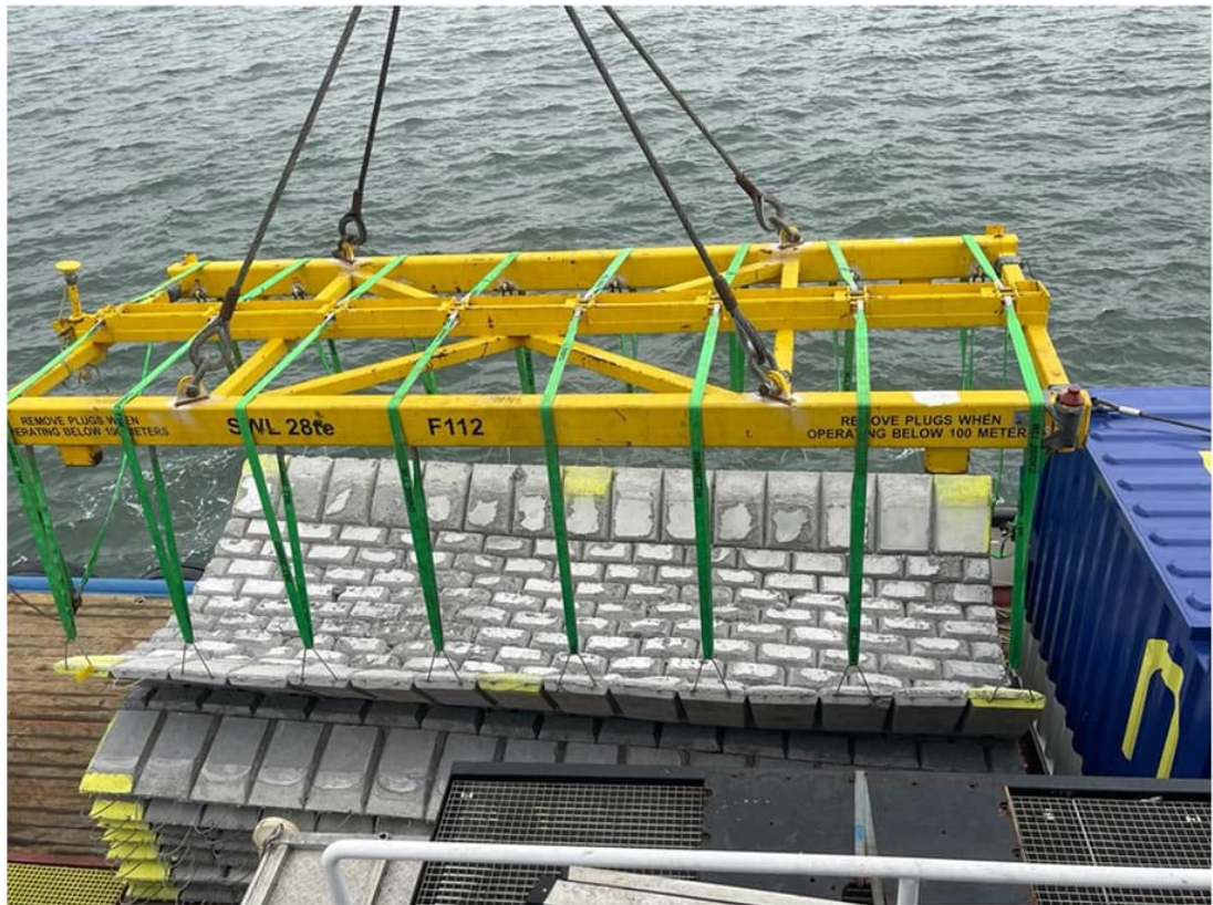
Figure 5-22 Concrete Mattress Prior to Installation
