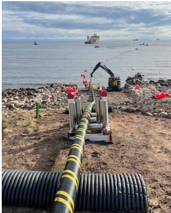
Figure 5-18 Example Images of Pull-In Setup
