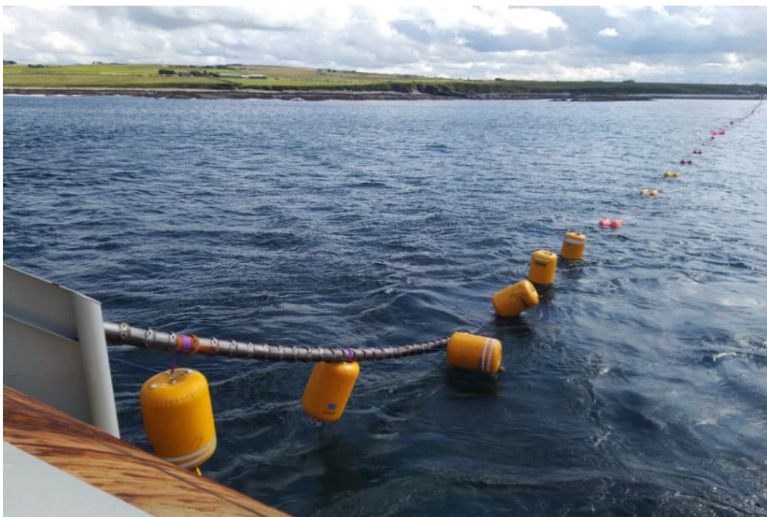
Figure 5-16 Cable During First End Pull-In Operations
