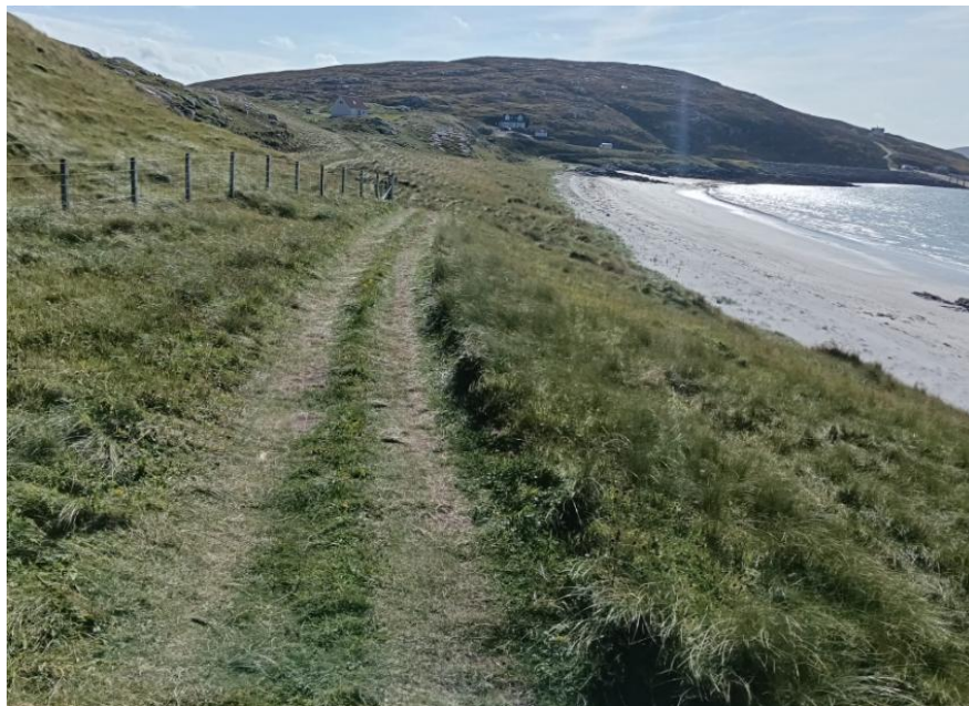
Figure 9 - Eriskay Access Track
