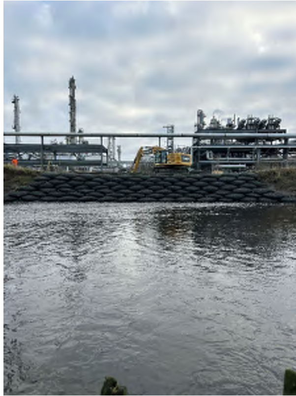
Figure 3: Completed rock bag installation.
