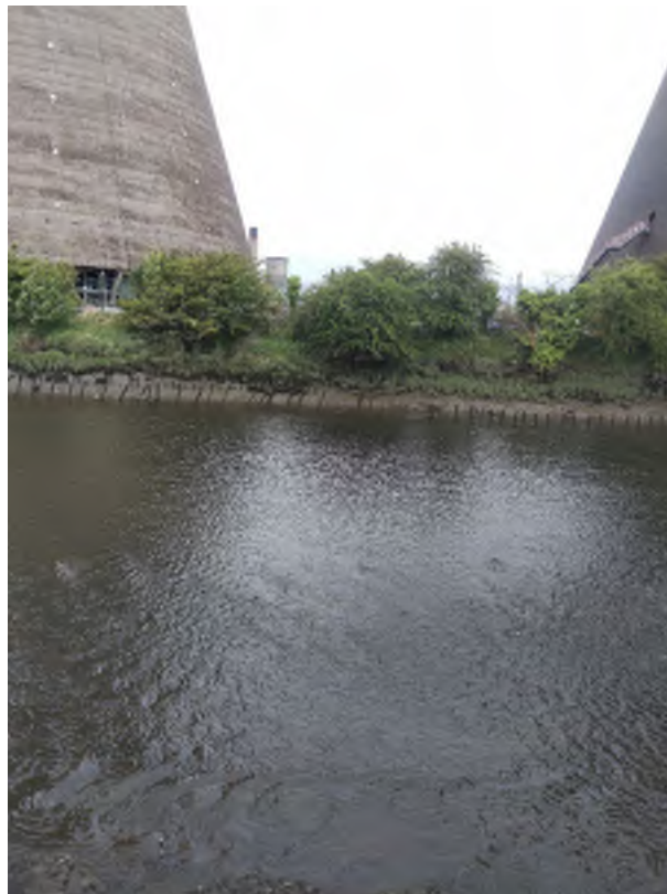
Figure 4: Adjacent Riverbank May 2025 – indicating no erosion
