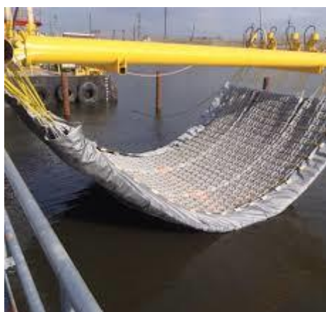
Figure 12. Scour protection concrete mattress
