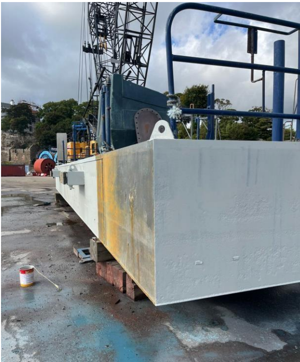
Fig-4 Thickness testing & Painting.
