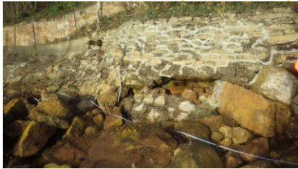
Large areas of washout, including erosion of previous bagwork repair.
