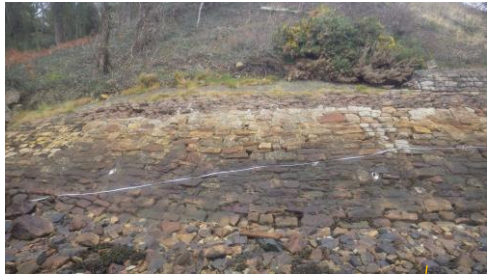
Erosion and washout of masonry and bagwork revetment face.
