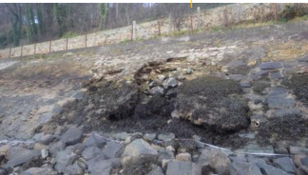
Large areas of washout, including erosion of previous bagwork repair.
