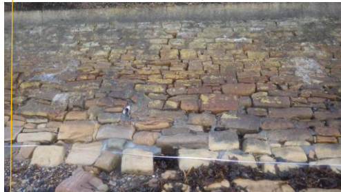
Loss of pointing across revetment face, loss of individual stones. Similar defects encountered on Sections 1, 3 and 5.
