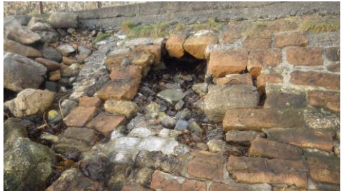
Washout and voiding near existing collapse with rip-rap repair.
