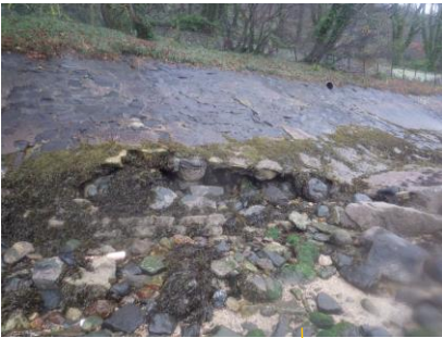
Erosion of revetment toe, and vegetation growth at crest of revetment.
