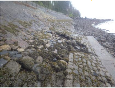
Erosion of revetment face and loss of existing bagwork repair.
