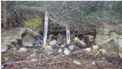
Erosion and undercutting of exposed soil slope beyond end of revetment.
