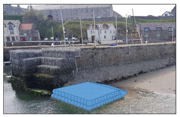
Stage 4: Remove material directly behind gabion baskets using the 20ton excavator
