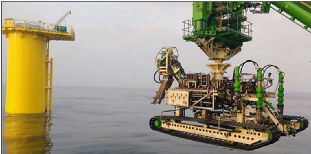
Figure 7-4: Deployment of a hybrid cable trenching tool
