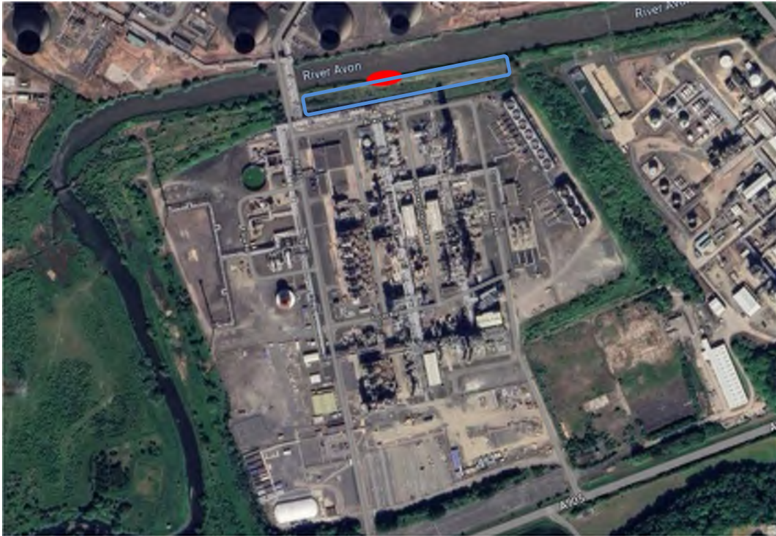
Blue box marking the approximate location of the haul road. The red circle indicating the approximate location of the temporary safeguarding rock bags.
