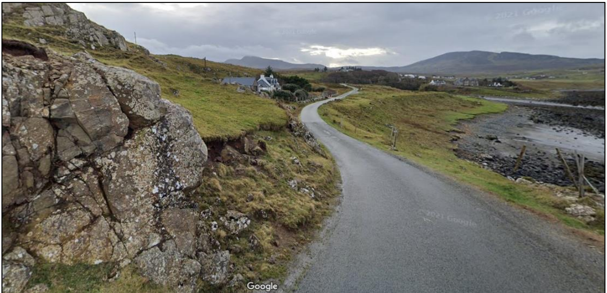
Plate 1: Looking west from road improvement location 7 to 5 (© Google Streetview)
