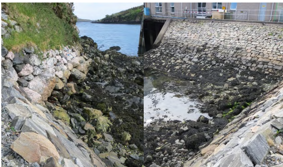
Photographs 6 and 7 Rock armour and seawall to east of ferry terminal
