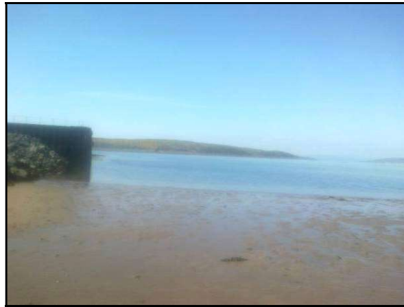
Photo 3: Area in front of existing quay to be dredged.
