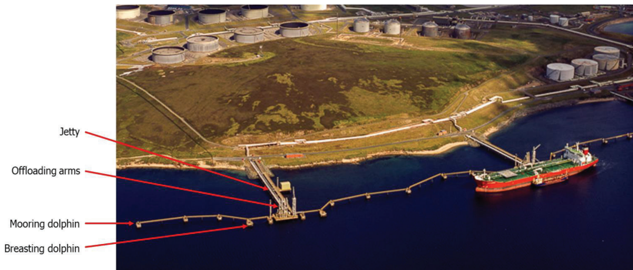
Figure 5-4 Labelled aerial photo of Sullom Voe Oil Terminal showing a similar jetty and typical jetty components. Source: Kent (2025c)
