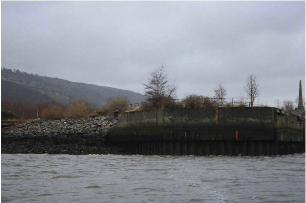
5) Western corner of sheet pile wall extending into inlet
