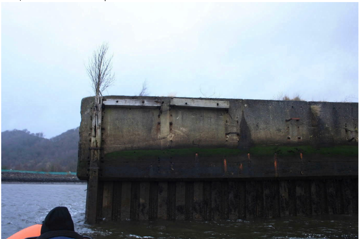
4) Western end of sheet pile wall
