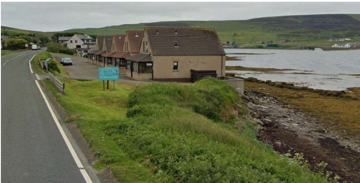
Pre development view of the site from the south east. A965 public roadway on the left. Road drainage 'offlets' in the foreground leading to a wide swale like verge.
