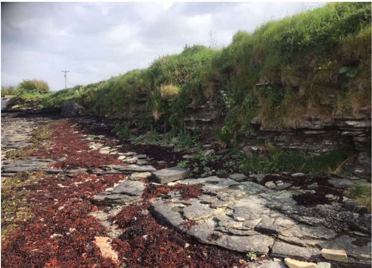
Natural shore profile immediately to the east of the proposed termination of the terraced stonework against the vertical bedrock cliff. Note the exposed bedrock backshore and near horizontal bedding
