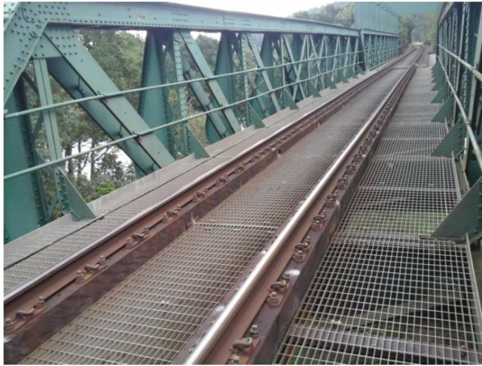
Photo 4: Track View - At Span 2 towards Low Mileage (11/08/21)
