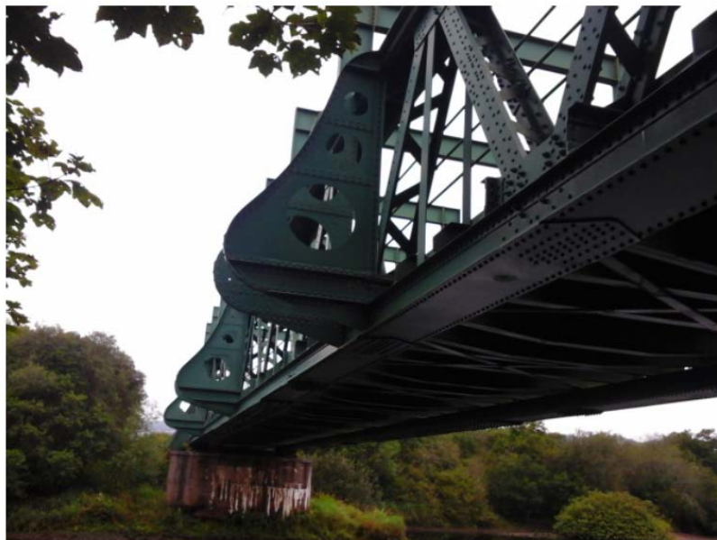
Photo 1: Downside Elevation from Span 1 (11/08/21)
